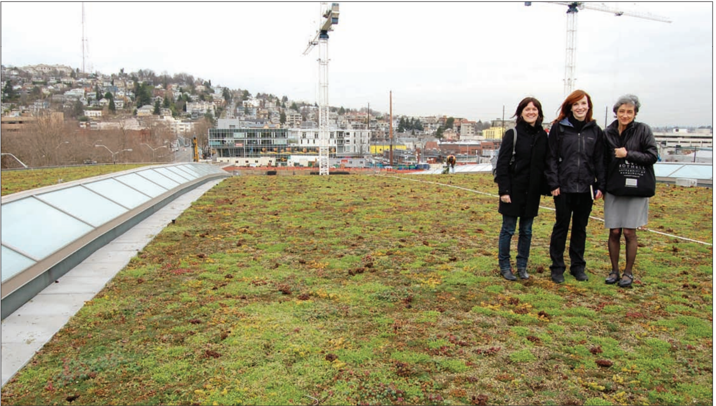
Amy Cragg and Shannon Nichol of Gustafson Guthrie Nichol, and Jeanne Iannucci of NBBJ, stand on the 60,000-square-foot green roof they all helped create.
